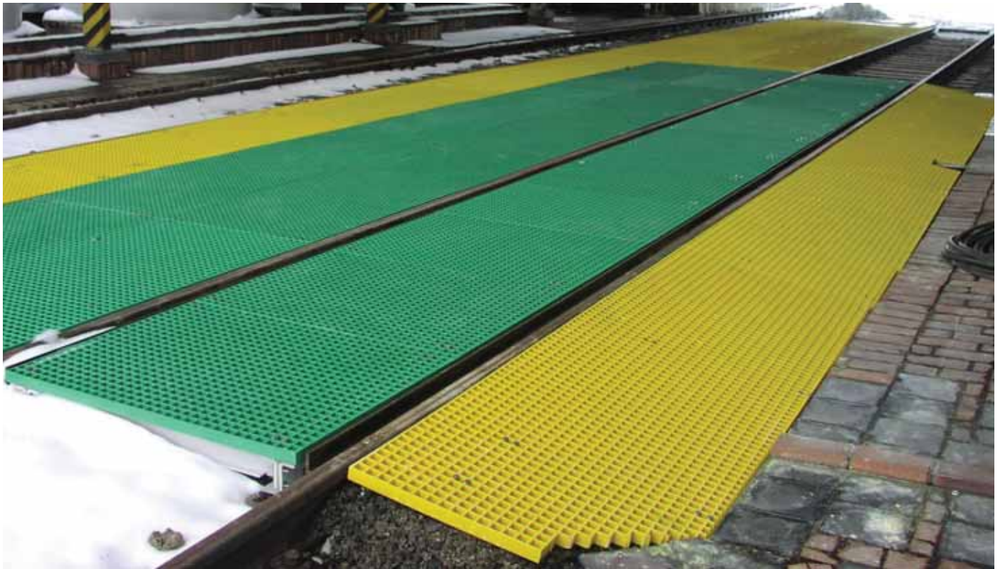
LOAD BEARING GRATINGS IN DUKOVANY NUCLEAR POWER PLANT DEPOT
