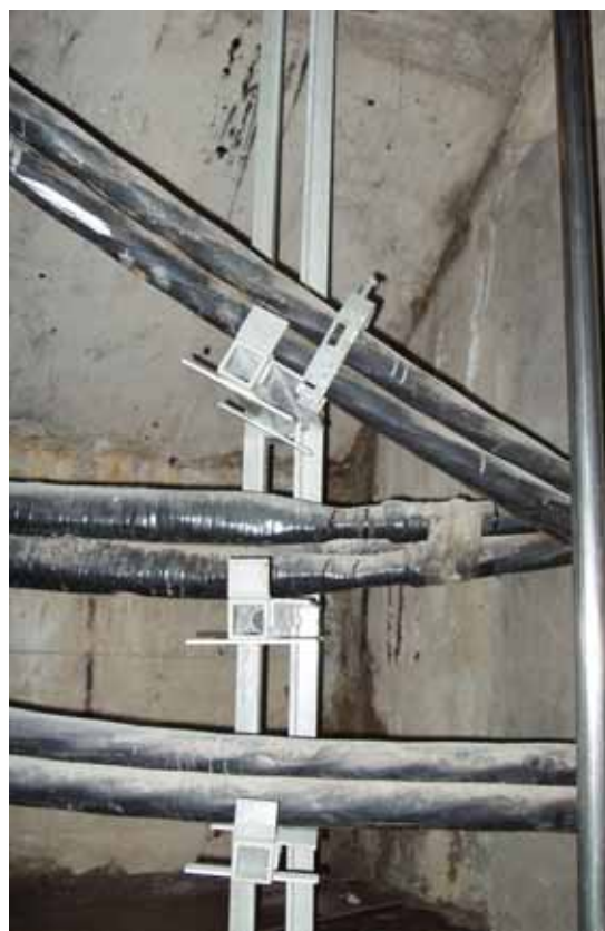
CABLE SUPPORTS WITH ADJUSTABLE BEDS – UTILITY TUNNEL IN PRAGUE, CZECH REPUBLIC
