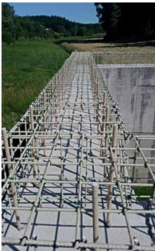
FRP COMPOSITE REINFORCEMENT, POLDER NEAR LUKA N. J., CZECH REPUBLIC
