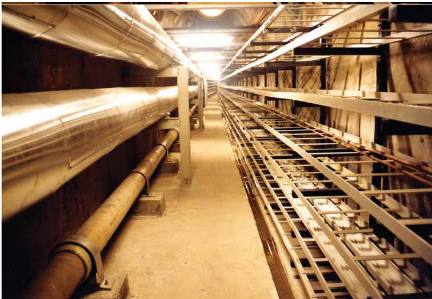
CABLE BRIDGES AND SUPPORTS – UTILITY TUNNEL IN DOWNTOWN OSTRAVA, CZECH REPUBLIC
