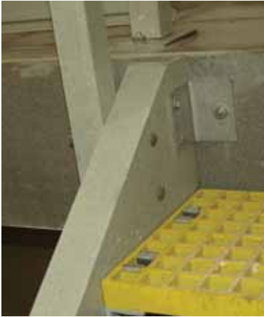
SUPPORT RAIL ANCHORING DETAIL
