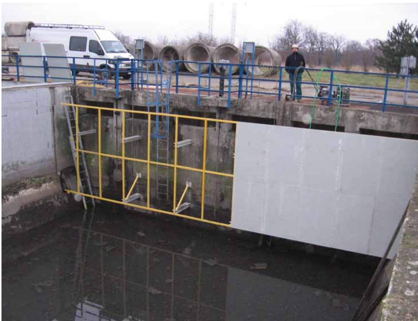
SCUMBOARD IN RAINWATER SEDIMENTATION TANK, PRAGUE, CZECH REPUBLIC
