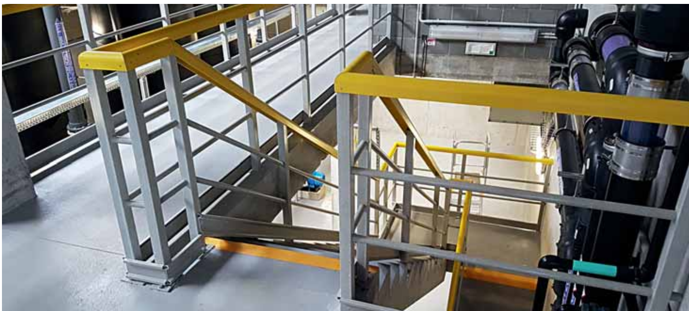
RAILINGS – TOP RAIL U 60.5 X 65/5 IN WASTEWATER TREATMENT PLANT, PRAGUE – ORDER VOLUME: 5.5 KM
