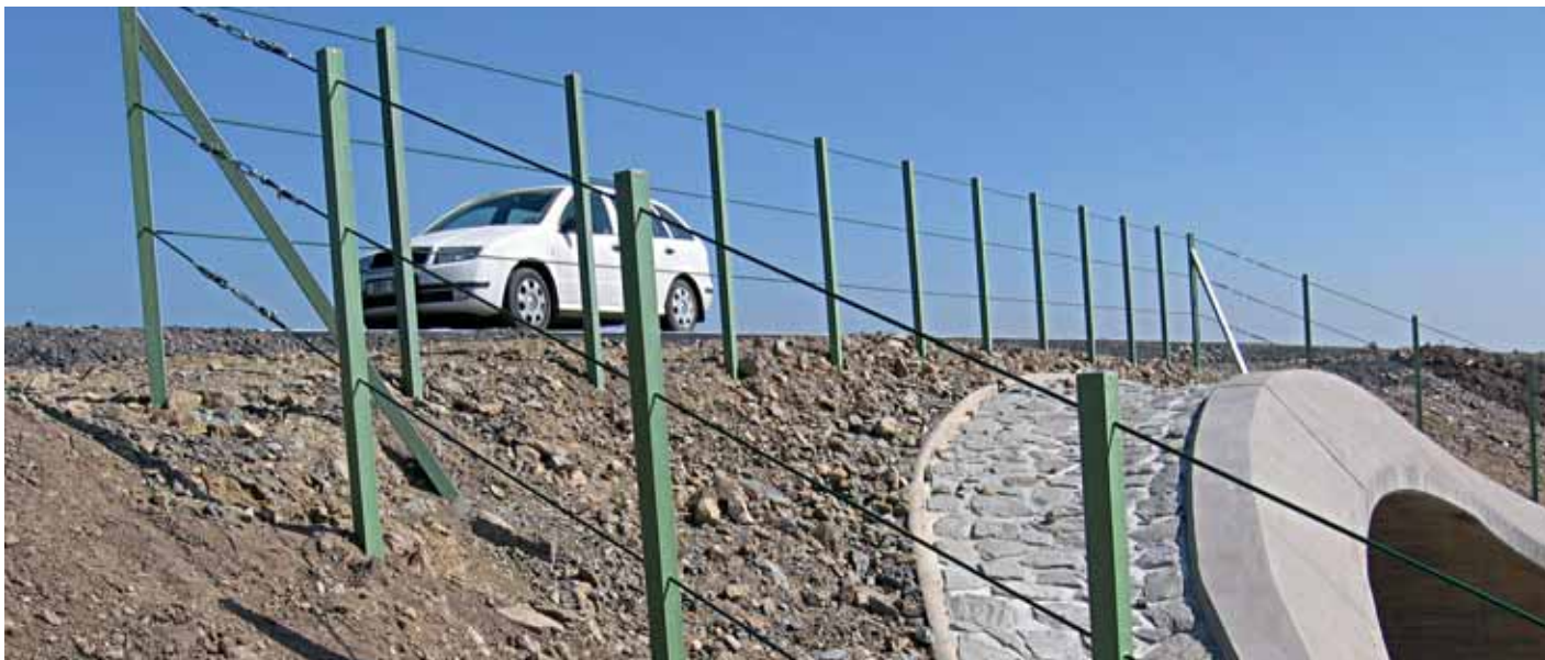
RAILINGS WITH HORIZONTAL STAINLESS STEEL CABLE, D8 PRAGUE
