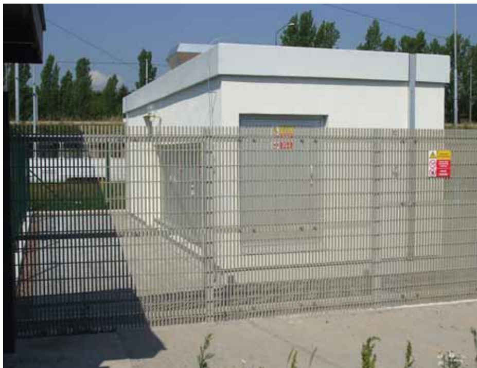
NON-CONDUCTIVE FENCE – MODŘICE TRANSFORMER STATION, CZECH REPUBLIC
