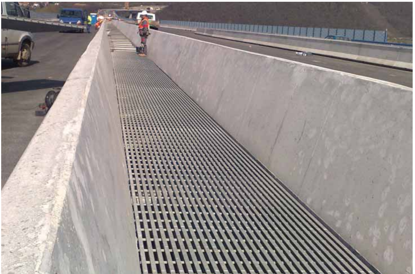
BRIDGE GAP COVER – MOTORWAY BRIDGE ON PRAGUE CIRCUIT HIGHWAY
