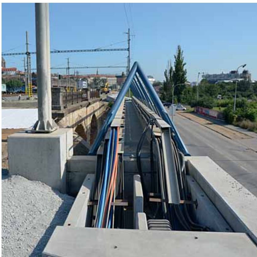
CABLE BOXES – UTILITY BRIDGE NEAR THE MAIN TRAIN STATION BRNO, CZECH REPUBLIC
