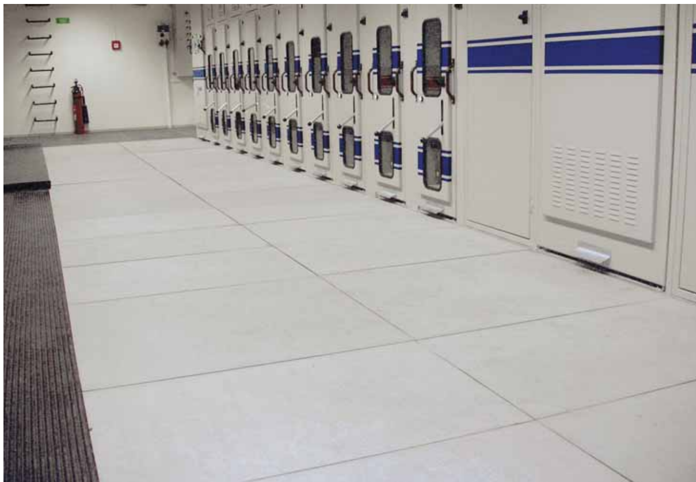
NON-CONDUCTIVE FLOOR – TRANSFORMER STATION IN BRNO, CZECH REPUBLIC
