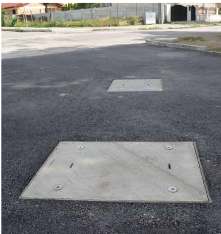
D 400 LOAD-BEARING COVER, FLOOD CONTROL CHAMBER – PEZINOK, SLOVAKIA
