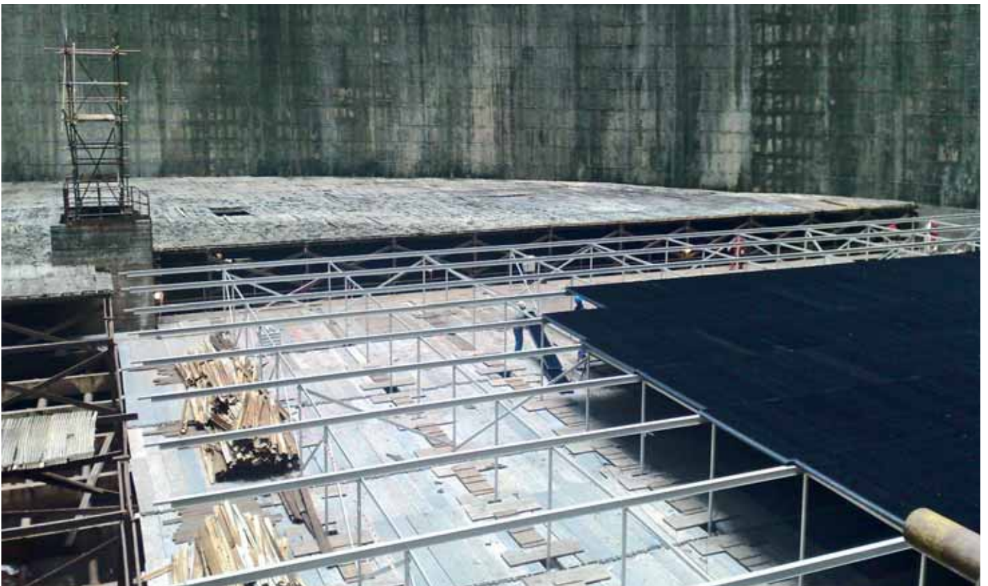
ELIMINATOR FRAMES IN DUKOVANY NUCLEAR POWER STATION, CZECH REPUBLIC
