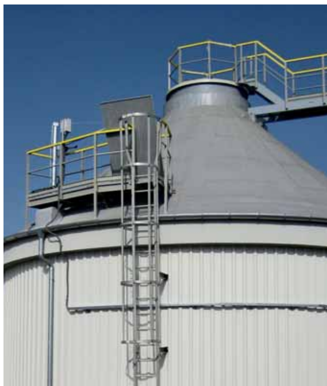
COMPOSITE LADDER WITH SAFETY CAGE – MODRA WASTEWATER TREATMENT PLANT, SLOVAKIA
